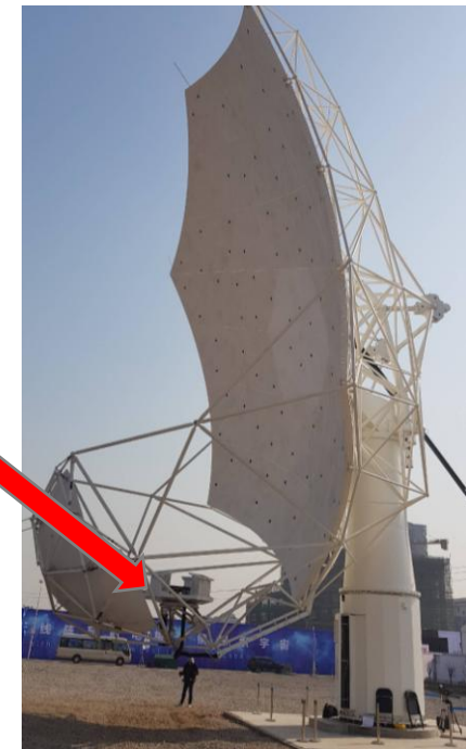
«SKA-P prototype, feed indexer and antenna structure (Shijiazhuang, China)
