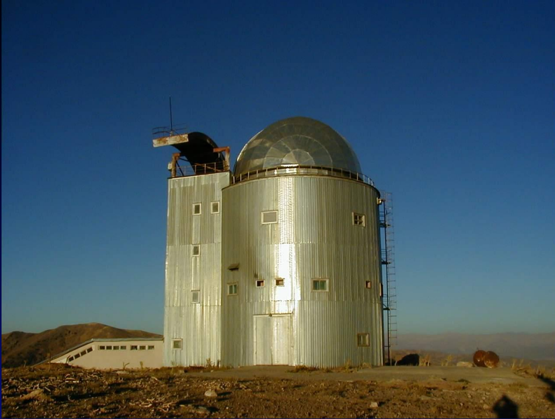
Tower of AZT-22
